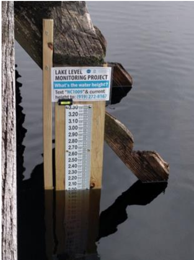
Water level Gauge
